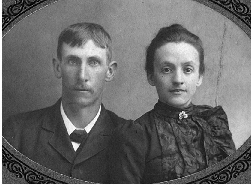
10. Sidi Hammet Ward (1873-1959) and Annie G. Wells (1875-1956)
