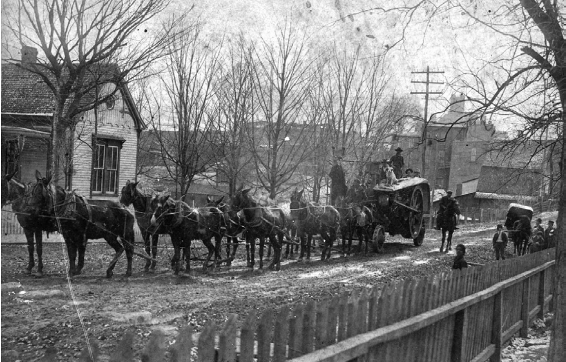
60. Mr. J.D. Ebert moving his cable tool drilling rig with a ten-mule team. J.D. was the father of Eldridge Ebert, who married Lucy May Ward. The view is on Washington Street looking west toward the courthouse in Glasgow, Barren Co., Ky. – January 1899.
