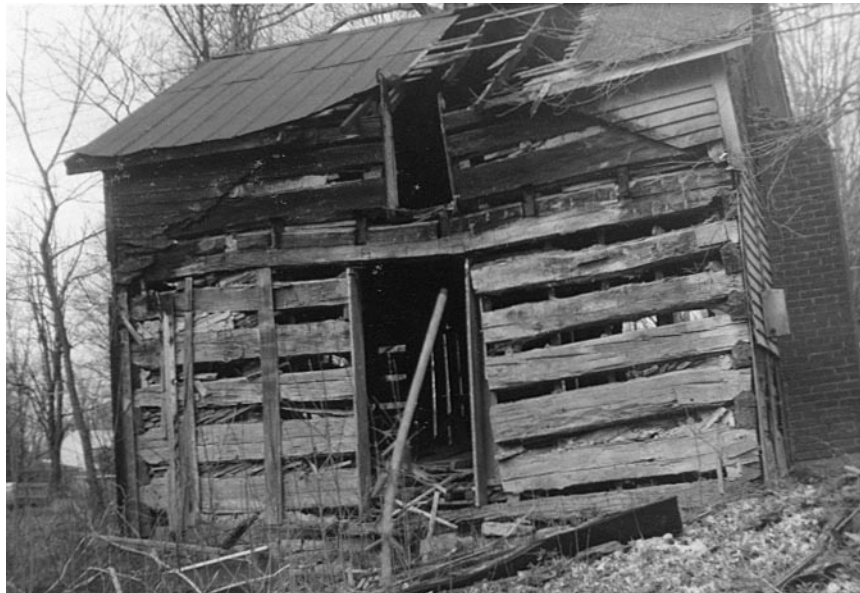
9. Rear view of the house showing the poplar logs exposed when the rear extension was torn away. The cabin was built about 1812 when John Nichols first settled in the area. Nothing remains on the site today except the little knoll where the house was situated and the spring that provided drinking water a short walk away.
