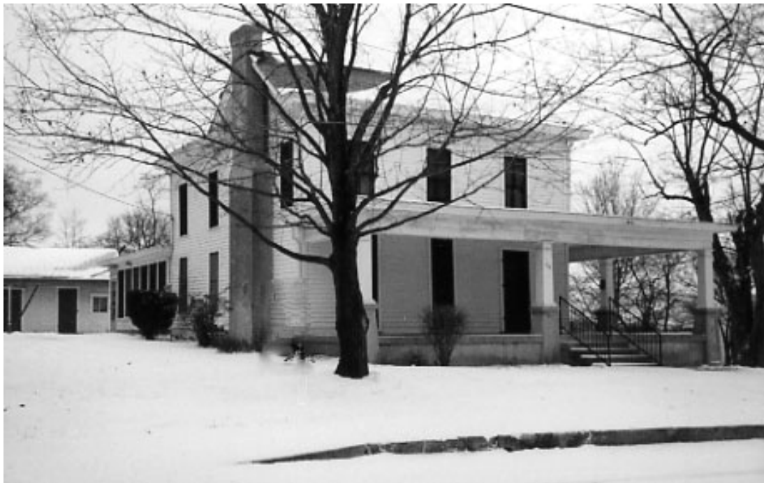
6. George P. McGee residence at Horse Cave in later years after structural renovations.
